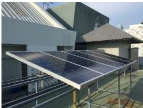
Figure 1. Terrace of the experimental building at KMUTT, Bangkhuntien campus.
